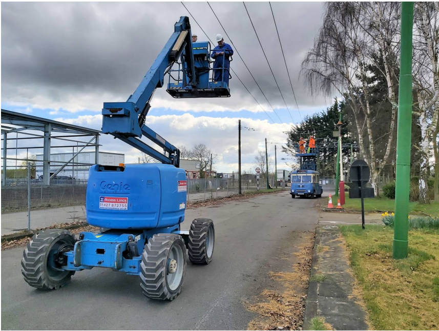
The Trolleybus Museum at Sandtoft's annual overhead line inspection is seen in progress on 15 March. As usual it was conducted by Andy Feather and Norman Hinchliffe and this year they were also instructing new trainees. The MEWP was on hire pending delivery of the machine that STCL has purchased. The overhead line was passed as fit for use, ready for the new season. [DG Chick]
